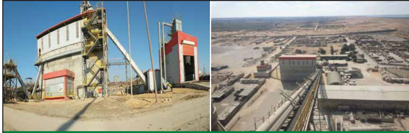
RDF System Installed on Line 3
