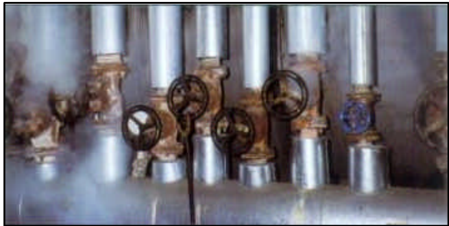
Steam pipe insulation in progress in the boiler house
