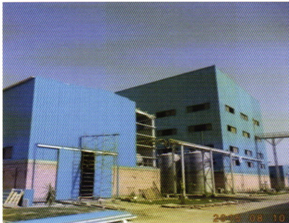
New Vacuum Plant
